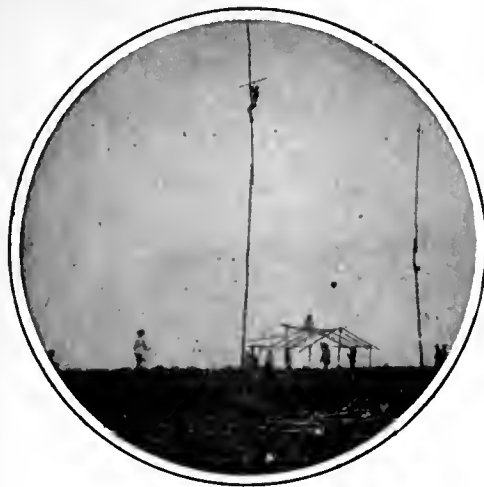
ERECTING WJS'S MASTS
